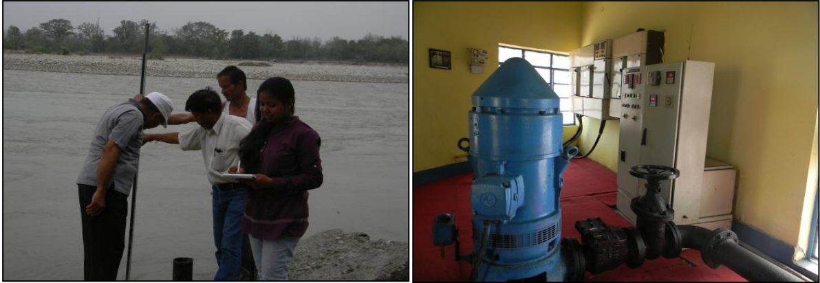
Plate2.Surface water level measurement and pumping unit of RBF well at Haridwar
